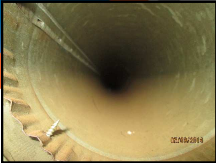
Supply branch before cleaning (shows significant effect of smoking in the home)
